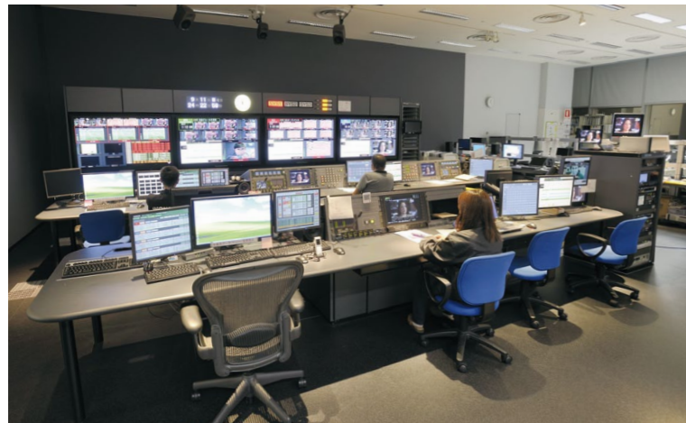
WOWOW's broadcasting center transmits radio waves to a broadcasting satellite via its uplink center in Tokyo.
